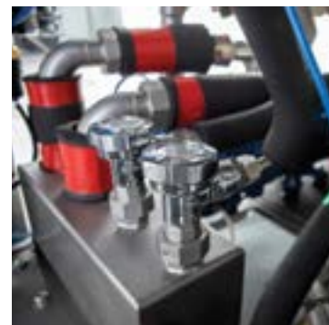
AISI 304 & AISI 316 piping design with connections & components
